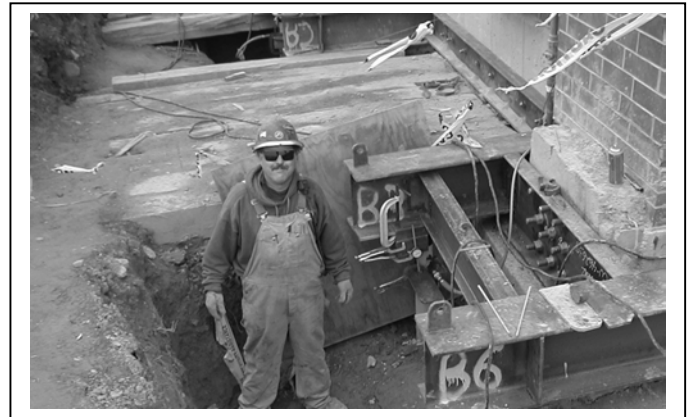
Fig. 5. View of completed piles and steel grillage.
